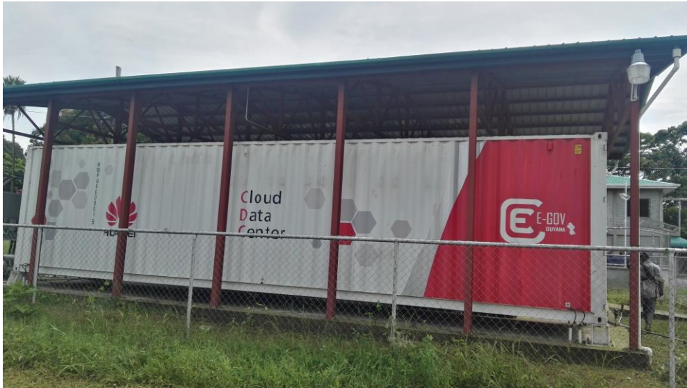
Image 232 - eGovernment unit's Cloud Service Infrastructure
