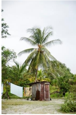
Image 43 - Pit latrine with slab (Region 4)
